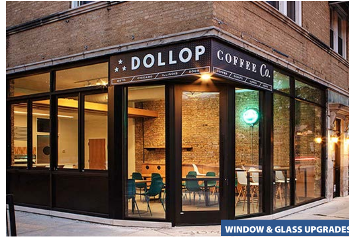
WINDOW & GLASS UPGRADES
